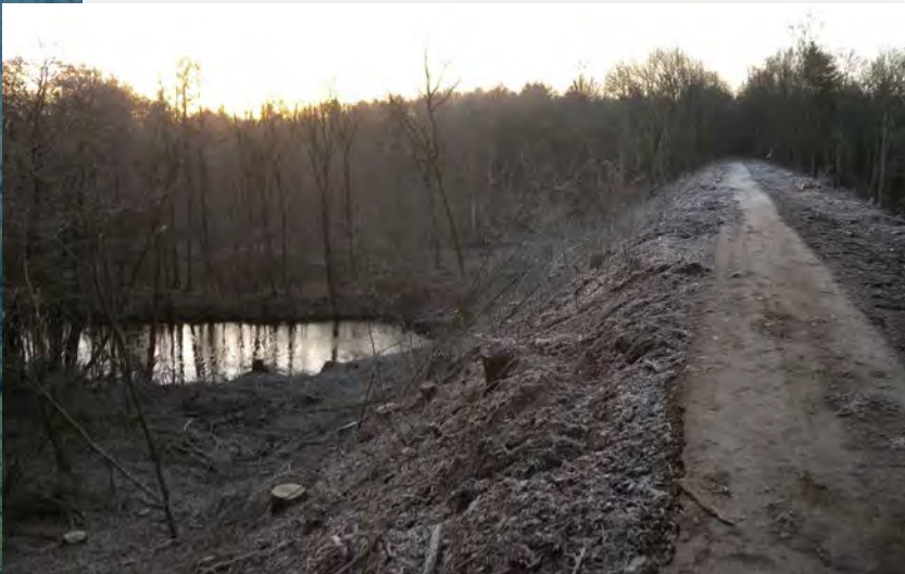
The embankment before excavation work commenced.
